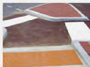
Kerbs, step and intersection pram ramps
